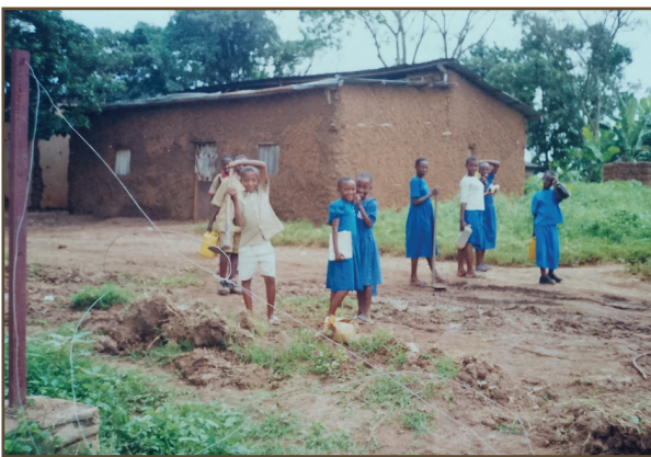
Kids from a neighbor school watch the bulldozers
